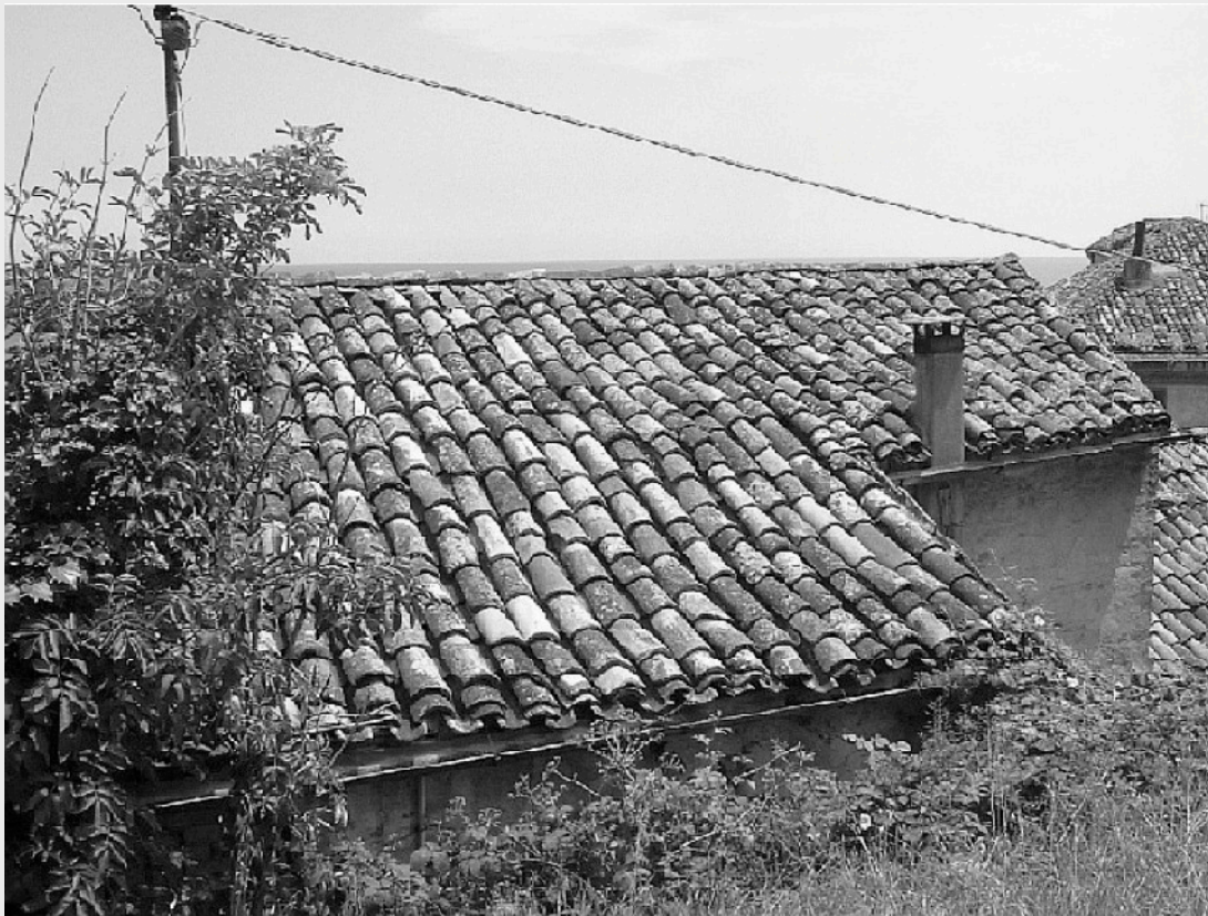
Fig.6.46 A vernacular Italian rooftop. The tiles, made by shaping clay around the tiler's thigh, is irreducibly full of affordance, and is therefore easy to empathise with.
